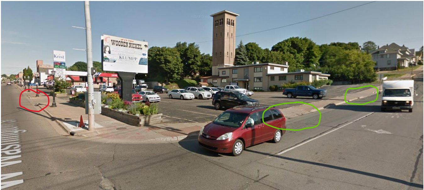
Figure 12 Redundant and Excess Driveways Reduce On-Street Parking and Sidewalk LOS
