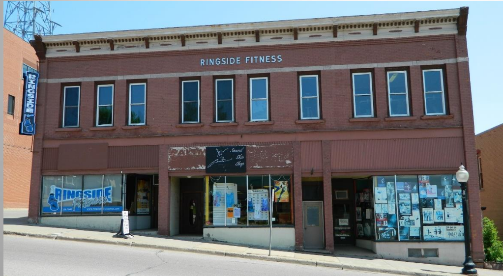
122 N. Third Street (Coles Bldg) Façade Improvement
