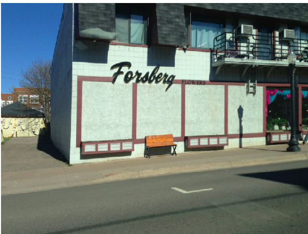
The Forsberg Flowers building is a mixed use building (retail with apartments above) and has a bench and boxes for flowers, but the identity of the business is somewhat muted.
