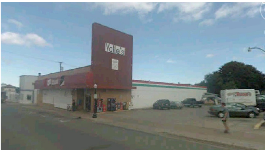
Existing view of Valle's Village Market and parking lot
