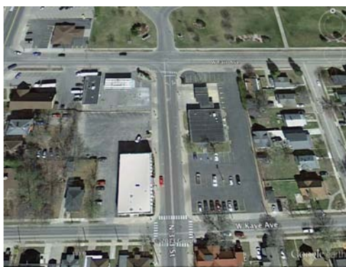
Aerial view looking north from West Kaye Avenue
