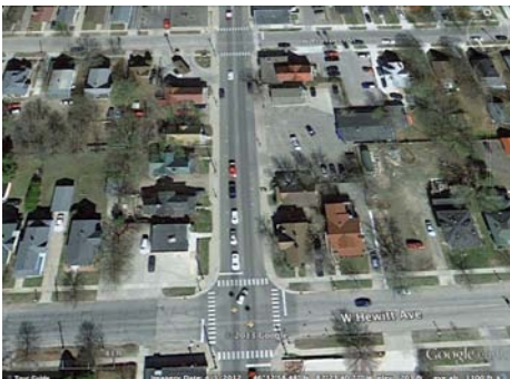
Aerial view looking north from West Hewitt Avenue
