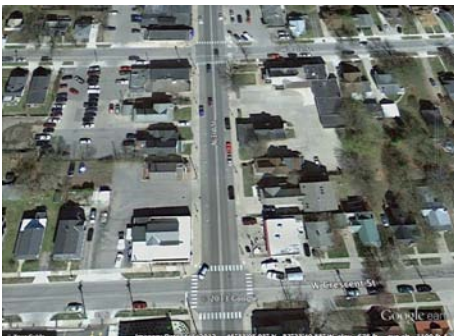
Aerial view looking north from West Crescent Street
