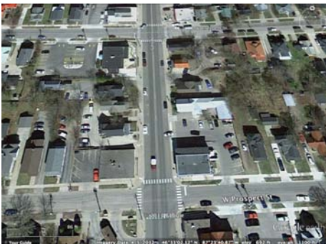
Aerial view looking north from West Prospect Street
