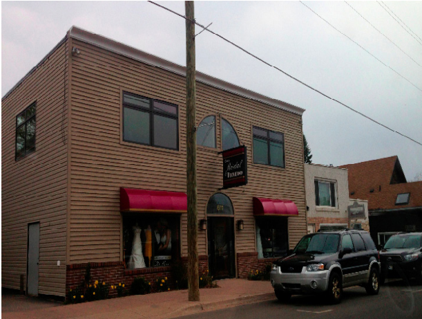
Dan's Bridal & Tuxedo is a good example of a true live/work building. A family owned business since 1974, it is a favorite of the community. The narrow strip of planting influenced the idea of a small setback on new buildings based on proposed Form-Based Code.
