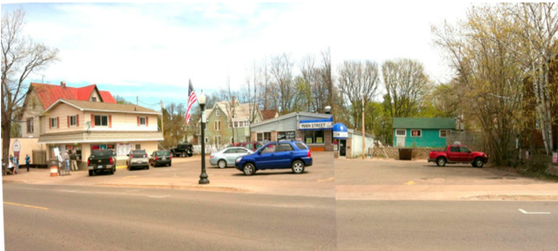
Existing view of parking lot next to Frosty Treats
