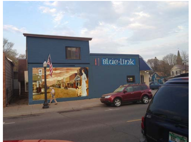
Storefront windows would be ideal, but in the short term, interest can be accomplished through a strong color surrounding a mural that indicates life.
